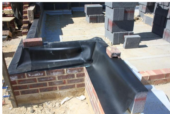
Visqueen Zedex DPC Corner Unit Application Example
