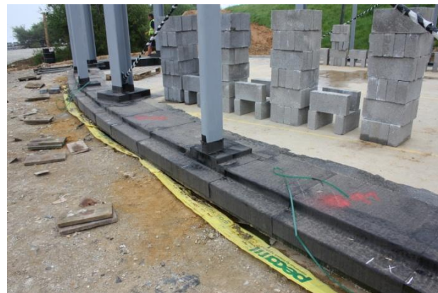
Visqueen TorchOn Tanking DPC applied to Steel Stanchions
