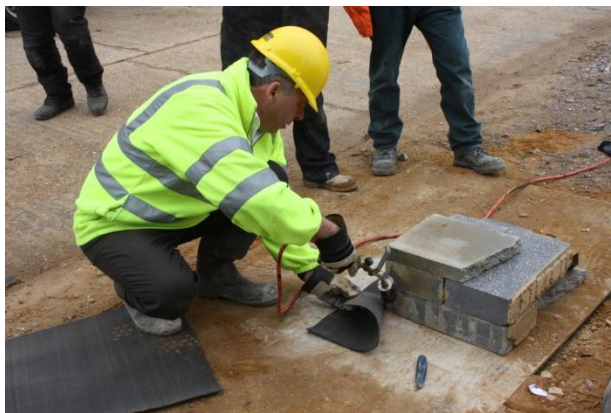
Visqueen TorchOn Tanking DPC Application Demo
